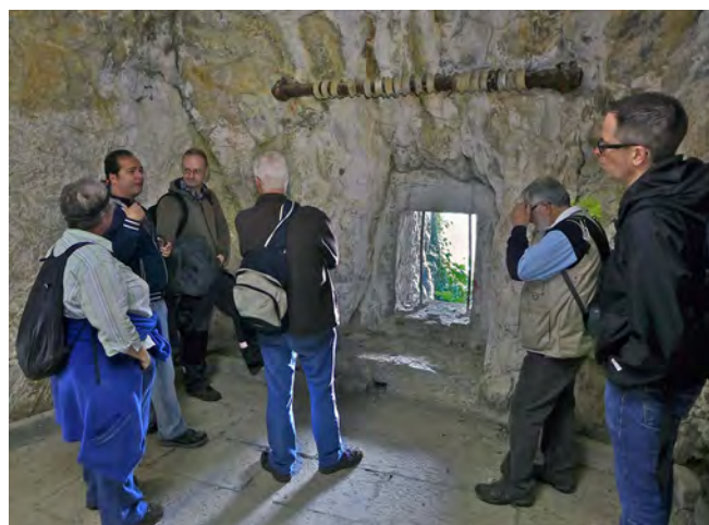
Carl explains the Lower Union Gallery gun emplacements. Note the rail for the splinter curtain
